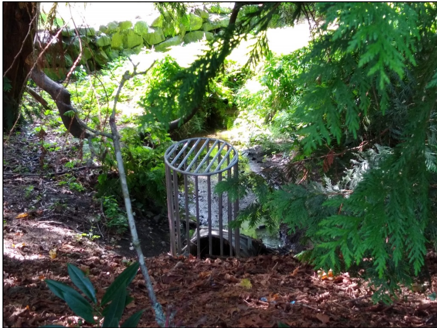
Figure 6. Photograph of Stream A taken from SE 33 rd Street.
